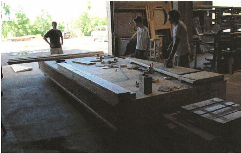
Figure 8: Borealis 3 Top Mold after Framing
