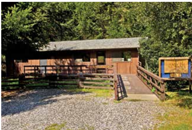
Accessible visitor center
