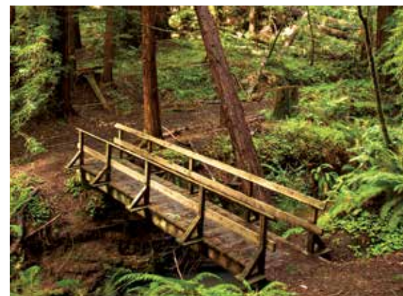
Bridge access over Butano Creek
