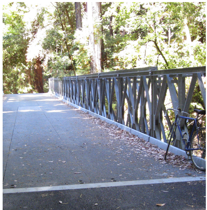
New Pescadero Creek bridge, 2010. Haul Road access.
