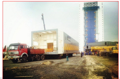
One of the umbilical towers still on the ground. Once installed on the launch platform, they will provide support of fueling, gas, air conditioning and power supply to the launcher. The VAB and the launch platform are seen in the background. (credit: Guangzhou Transportation Co. Ltd.)
