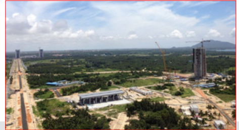
View from the top of the CZ-5 tower. At the left of the picture, there are two vertical assembly buildings (VAB) in the distance. At the right of the picture is the launch tower for CZ-7. The two VABs and two launch towers are linked with tracks. (credit: Chinese internet)
