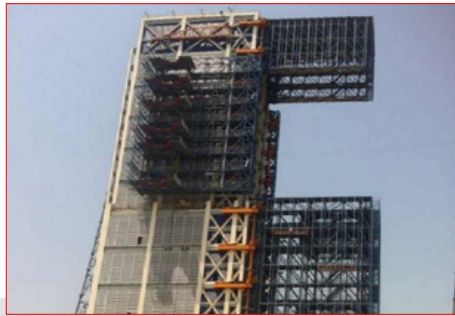
Full view of the CZ-5 launch tower, taken in early 2014. The tower had almost been completed when the photo was taken. Note, that there is no crane at its top, which is the first time for a Chinese launch tower. (credit: Chinese internet)
