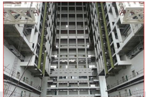
Interior view of the vertical assembly building. (credit: Chinese internet)
