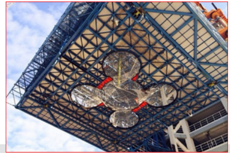
Close-up view of the bottom-most platform when closed, looking from the ground. The space for the 5 m diameter core stage and four strap-on boosters are seen at the centre of the platform. (credit: Chinese internet)
