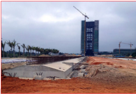
The tracks from the vertical assembly building to the launch pads under construction. The picture shows that the bed for one of two tracks has been almost completed. The vertical assembly building and another track are visible in the background at the left of the picture. (credit: Chinese internet)
